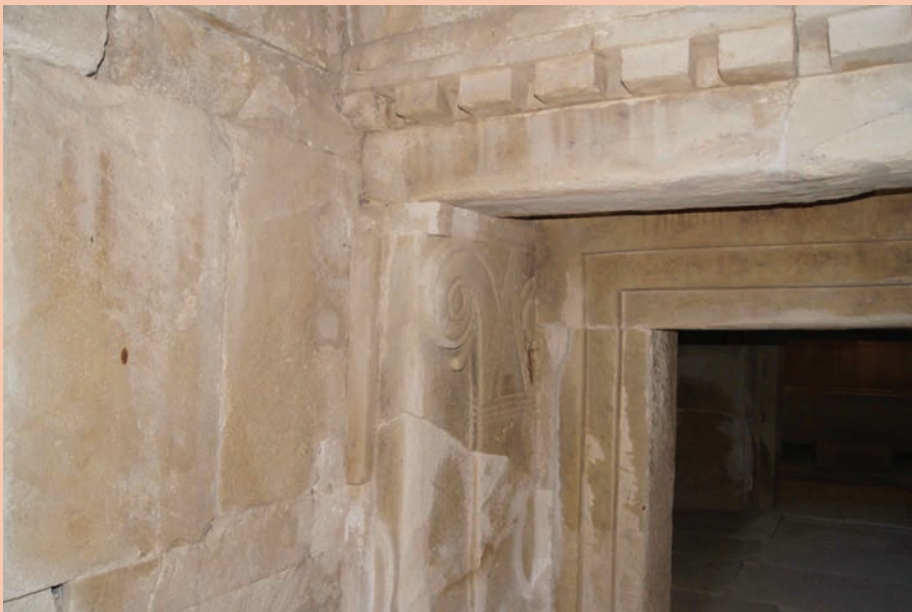
FIG. 15 Entrance of chamber tomb (Tomb 5) at Tamassos (Cyprus, seventh–early fifth centuries BCE). Flanking the entrance to the tomb are two almost identical volute capitals, rendered in relief on flat pilasters. The entrance itself is characterized by a stepped or recessed frame. Above the lintel are the ends of imitations of rectangular wooden beams. Virtually all elements in the grave imitate woodwork and timber construction. (Photo by Rjdeadly, CC BY-SA 4.0 [ https://creativecommons.org/licenses/by-sa/4.0/ ].)
