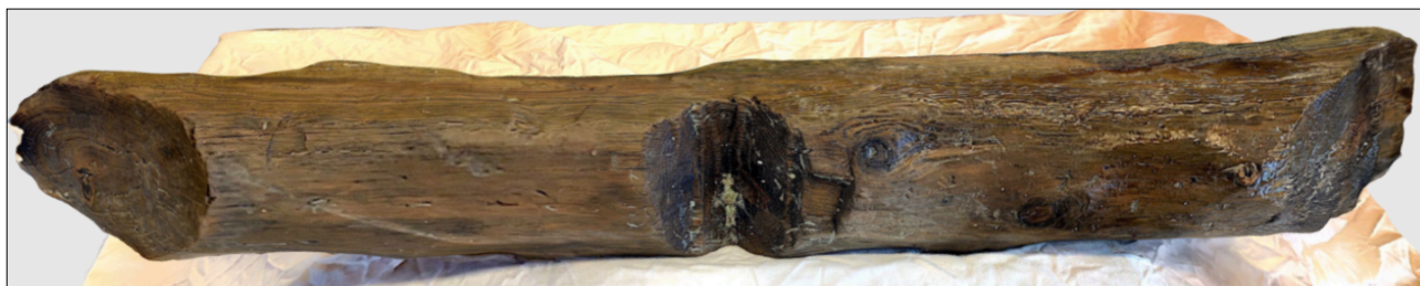
Fig. 5. 3D model of the top of a gable from a timber joint building, salvaged from the Bulwark by me in 2022. The roof angle here is 32 degrees. The building was thus built according to a traditional geometric formula, called 1/3-gable, where the height of the gable was 1/3 of the base width of the building. The formula was commonly used before the protractor was introduced. Note also the ax cut for the ridge in the middle, where a chop ax with a slightly convex edge of small dimensions was used. With the cut marks it is possible to reconstruct the ax. On the underside of the log there are recesses for the ends of the side beams, which can be used to interpret the roof construction. Model: Peter d'Agnan.
