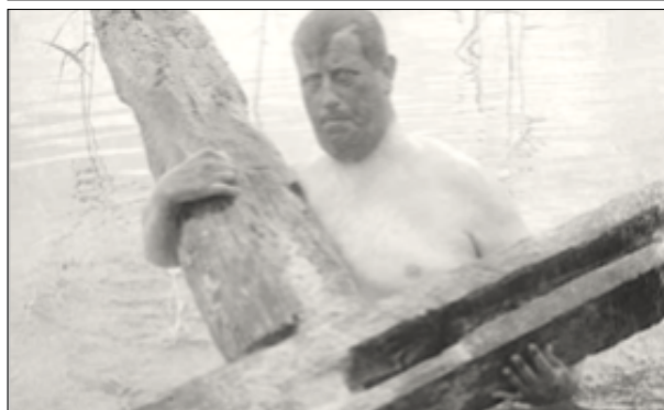
Fig. 2-3. Arvid Zetterling and his friend Lennart von Post with salvaged building parts which through craft science and building analyses, can provide new knowledge of importance to the understanding of the development of wood culture. Here we see Arvid (on top), with a gable in a timber joint construction that can tell us about the size of the house.
